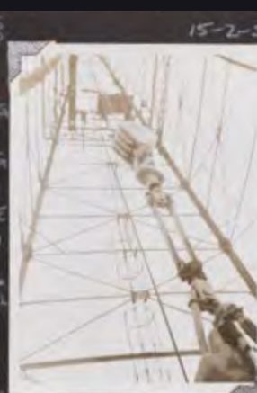
TWO VIEWS LOOKING UP AT THE MAIN DRILLING GEAR FROM THE WORKING PLATFORM SHOWING THE LARGE PULLEY BLOCK AND THE STEEL LADDER UP TO THE 85FT. PLATFORM.
